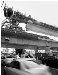
Last year's winner: The Caulfield to Dandenong Level Removal Crossing Project
