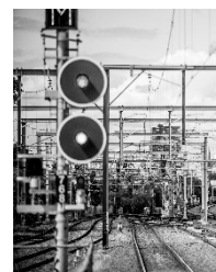
Last year's winner: Uninterruptible Power Supply For Melbourne's Railway Signalling Network
